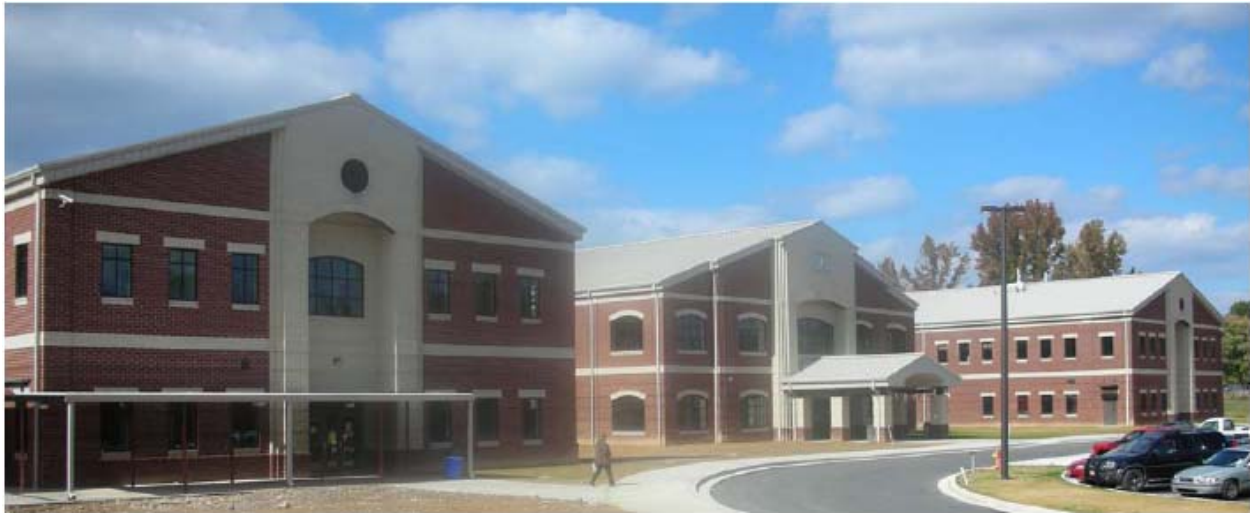
Figure 4: Main Classroom Buildings at Pepperell High School
